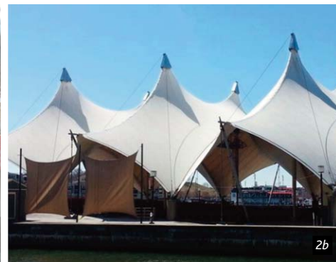
Figure 2a/b. Two different approaches to design the support of a membrane.
