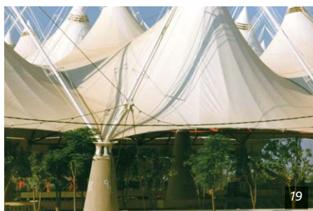
Figure 19. El Palenque: side view. Note the radial, valley and edge cables.
